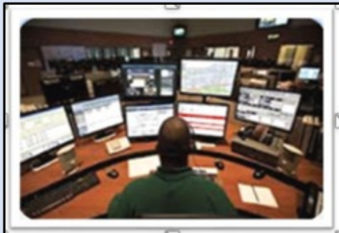
Integrated Command & Control Centers
